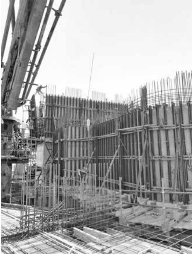
Water reservoir - Algeria
